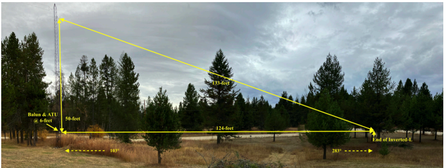
Tower, tower-stand-offs and Inverted-L antenna.
